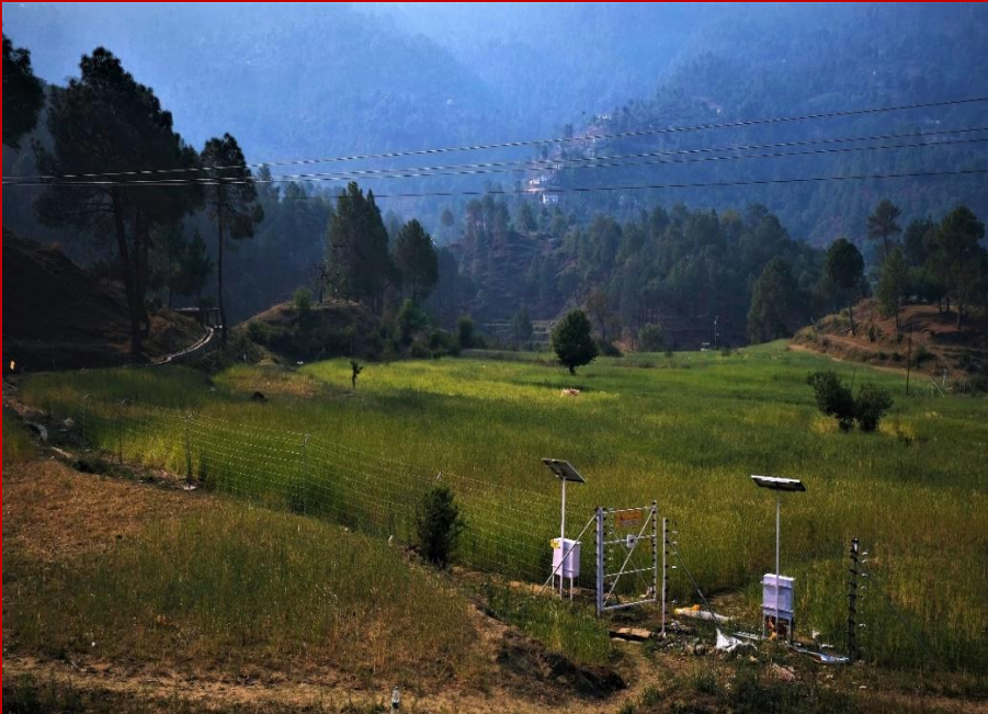
SOLAR FENCE INSTALLED AT VILLAGE PATIYA
